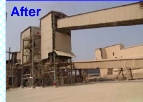
Sulphur Conveying System (SAP)
