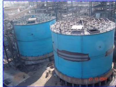
Construction of new Phosphoric Acid Storage Tanks
